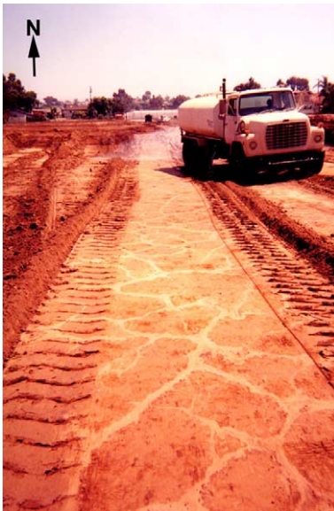
Fig. 15. A horizontally-graded terrace surface at Carlsbad, California (46.32 m el. MSL) exposing polygonal-shaped, “reticulated” multi-colored sand-filled features. Note: Vertical cuts of these same polygonal features expose numerous, adjacent, coalescing, upward-fining sand dikes demonstrably injected from below and not the result of surface infill.
